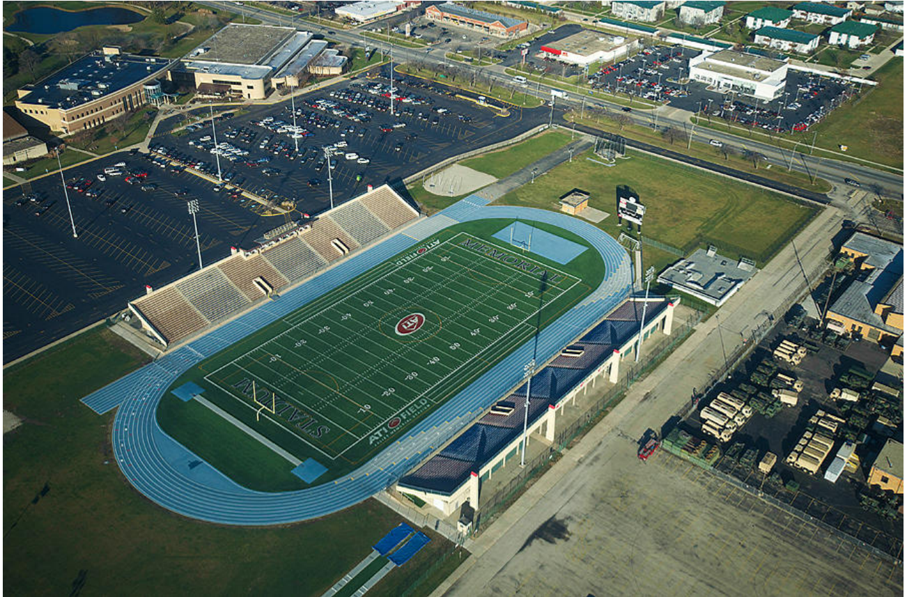
Joliet Memorial Stadium
